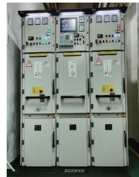
Shore power connection distribution panel
