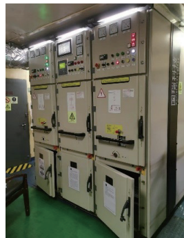
Shore power connection distribution panel
